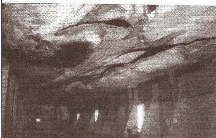
THE DAMAGED UNDERSIDE OF THE VESSEL, WITH THE LONGITUDINAL TEARS RUNNING FROM FORWARD TO AFT, PRIOR TO REPAIRS BEGINNING.
